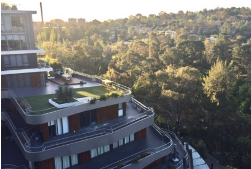
Figure 7.8: A children’s “play space” made of artificial turf installed on one of the largest terraces of Eden in Acacia Place, November 2017. Photo: L. Dorignon
